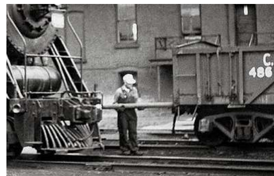
A push pole in use, between a steam locomotive and a gondola car. From an image by L.G. Gibson via Industrial Scenery online.
