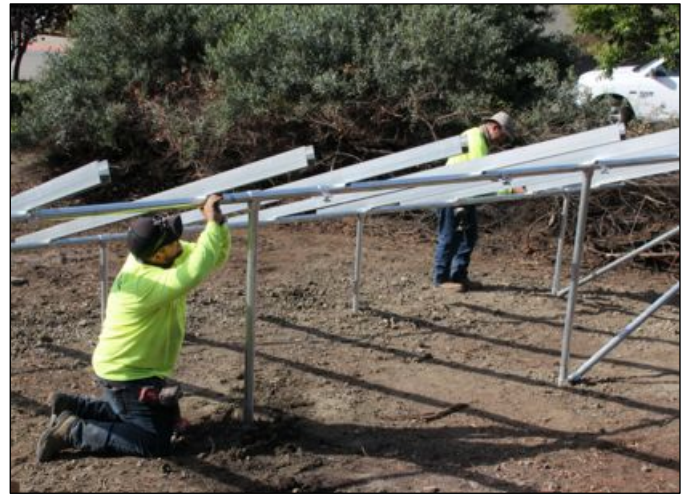
Bland workers assembled the frame (above) and attached the panels, each three feet wide and six feet long (below). Three photos by Gary See
