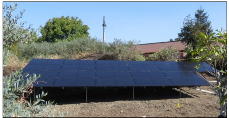
Above, the panels as seen from neighboring property to the south. The Freighthouse roof is visible in the background. See page 10 for more construction photos.
