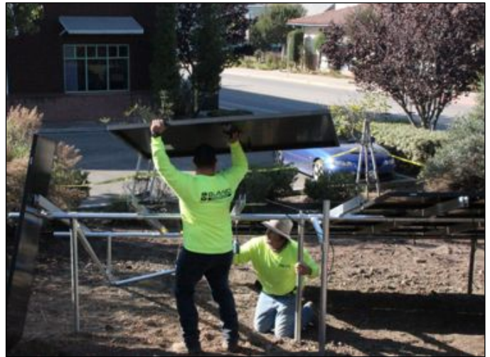
Bland workers assembled the frame (above) and attached the panels, each three feet wide and six feet long (below). Three photos by Gary See
