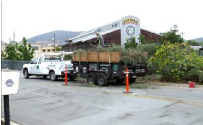
In early October, Dan's Landscaping workers cleared the densely overgrown site across from the Freighthouse.
